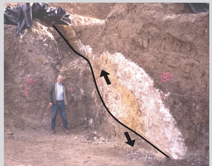
Figure 2B. View SE at thrust fault exposed in 2003 excavation. Fault thrusts Miocene marine shale (right) over Pliocene and Pleistocene non-marine gravel (left). Location of photo indicated in Fig. 2A.
