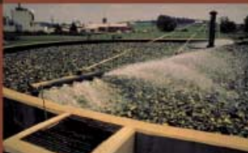
(Left) Trickling Filter at old Horse Cave Sewage Treatment Plant. The poorly treated effluent was discharged into caves and sinkholes upstream from the city of Horse Cave.
