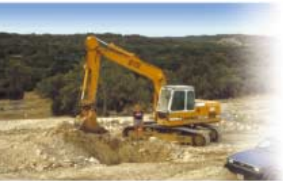
Fig. 49. A road being built over and sealing a cave runs the risk of collapse and problems with water quality and quantity.
