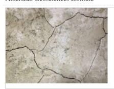
How do pyrite and pyrrhotite damage building foundations? American Geosciences Institute
