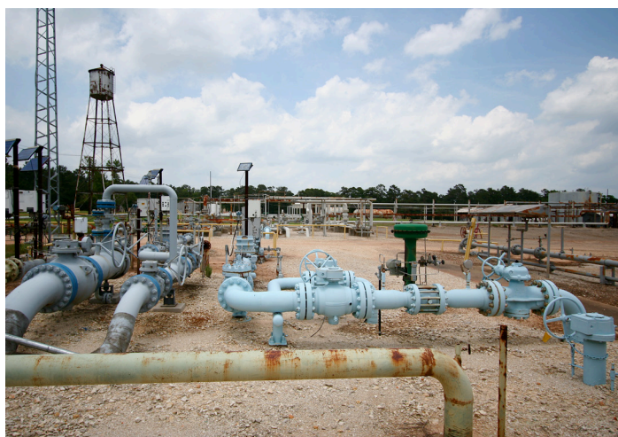
Natural gas infrastructure includes a large number of valves and connectors, such as at this gas processing facility in Montgomery County, Texas. Components such as these may be sources of gas leaks. Image credit: Roy Luck, Flickr. 12
