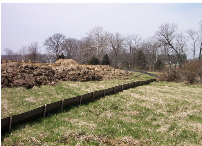
Plastic fencing to control soil erosion and stormwater runoff at a construction site. Image Credit: U.S. Environmental Protection Agency. 30
