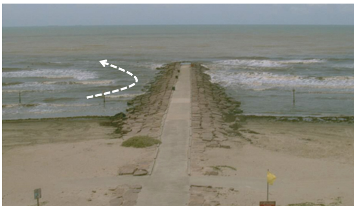
Galveston Island, Texas. Photograph shows a rip current on the left side of a groin. Beach access points are located at the center of each groin, and two signs mark the no swimming zone on each side. Image credit: Modified from Brannstrom et al. (2014). 8
