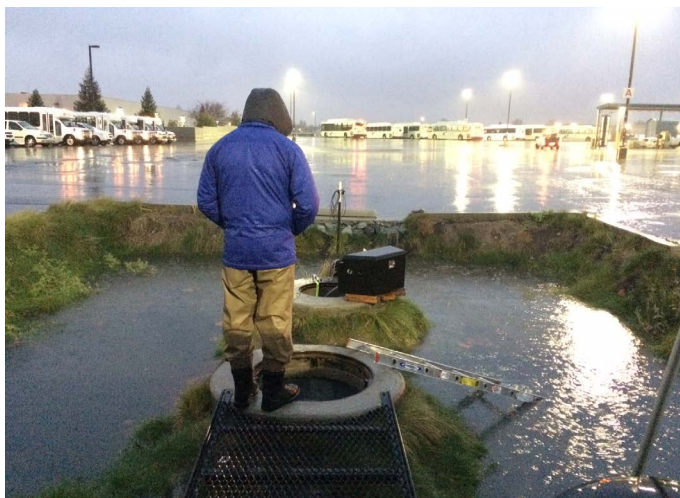
A vegetated pretreatment feature (grassy swale) with dry well in center. Image Credit: California Office of Environmental Health Hazard Assessment
