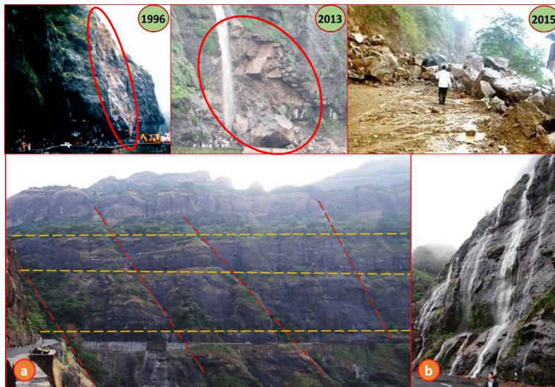
Figure 1: Major rockfall incidences occurred during the monsoon in 1996, 2013 and 2015 along Malshej Ghat section of NH-222, Maharashtra, India
