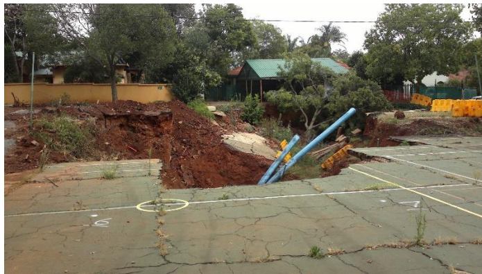
Figure 1: The Pretorius Street sinkhole shortly before commencement of rehabilitation.
