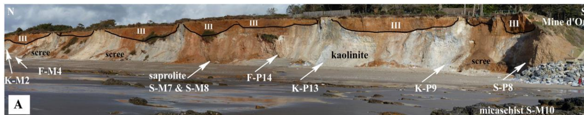
Figure 1: 500 m long, ~15m high coastal cliff, north of La Mine d'Or beach entrance, where micaschist is cropping out on the shore, saprolite is located at the cliff toe in different patches and the white kaolinite zone is cropping out in a relatively continuous way with a thickness of about 5–10 m. The top of the kaolinite zone is crosscut by an unconformity surface covered by Miocene to Pleistocene red clastic sediments (III) and Quaternary deposits. S–M#, K–P# and F–M# are locations of analyzed samples.
