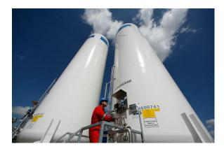
Two tanks for intermediate storage of  $CO_2$  with a capacity of 50 tons each were used during the operational phase (2008 – 2013) (Photo: GFZ).
