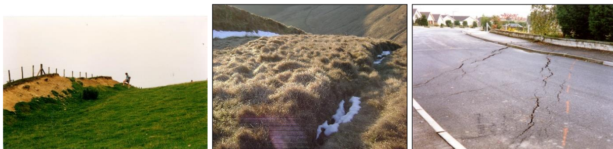
Figure 1 Variations in fault scarp morphology: (Left) Uphill facing, linear, fault scarp above the crest of Troedrhifwuch landslide, South Wales, UK. (Middle) Two parallel scarps, Tableland Fault scarp, South Wales, UK. (Middle) Small graben, Derbyshire, UK.
