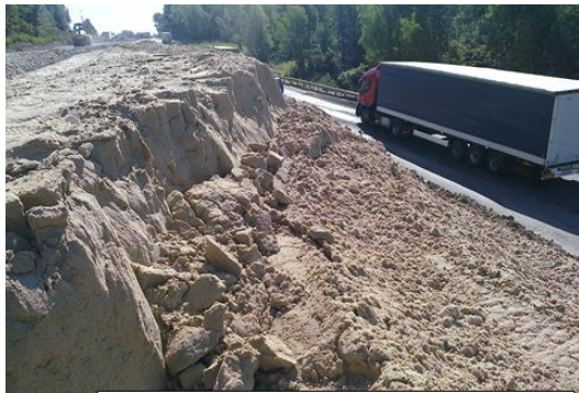
Fig. 1. Landslide crack on the embankment.
