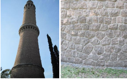
Figure 1 Colonia del Sacramento Wall
