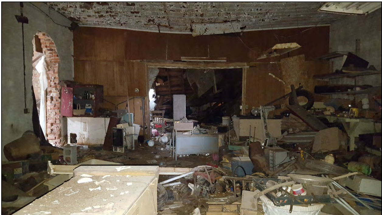
PHOTOGRAPH 12. Interior of middle room of Former Auto Repair Garage. Note assorted refuse and debris. Note sagging ceiling and water-damaged walls. View of collapsed rear room through opening in rear (western) wall of middle room.
