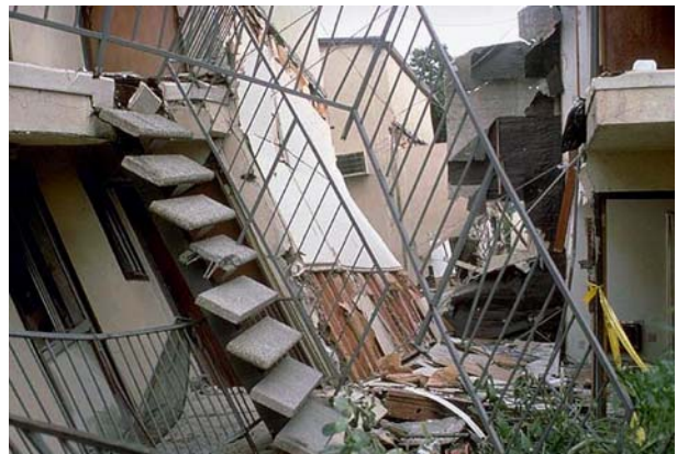
Collapse of apartment building over garage in Reseda following the 1971 San Fernando earthquake.
