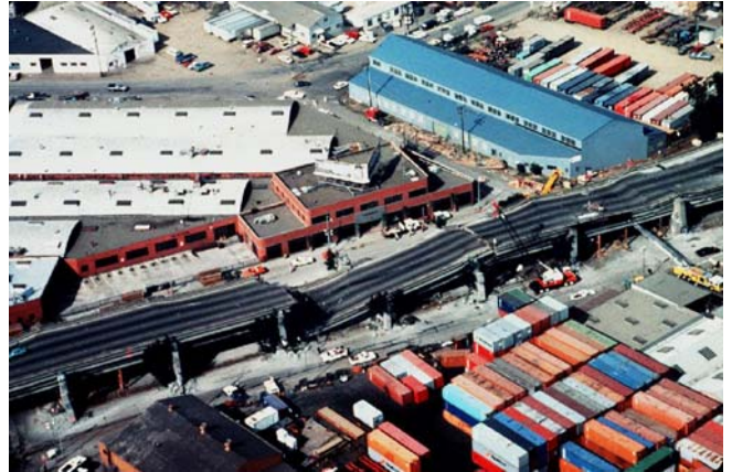
Collapsed Interstate 880 in California
