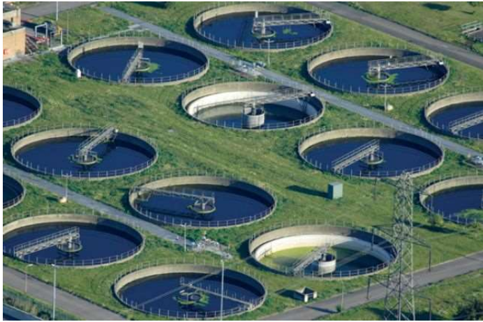
Figure 10. Water-processing plant. Credit: iStock
