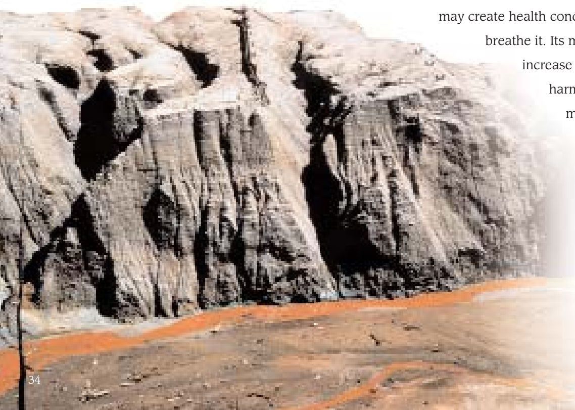
Fig. 20. As this small stream in Colorado erodes the mill tailings pile, it releases oxidized metal-bearing minerals into sediments downstream. The steep gray bank of unoxidized sulfide minerals shows characteristic layering that develops as tailings are deposited.
