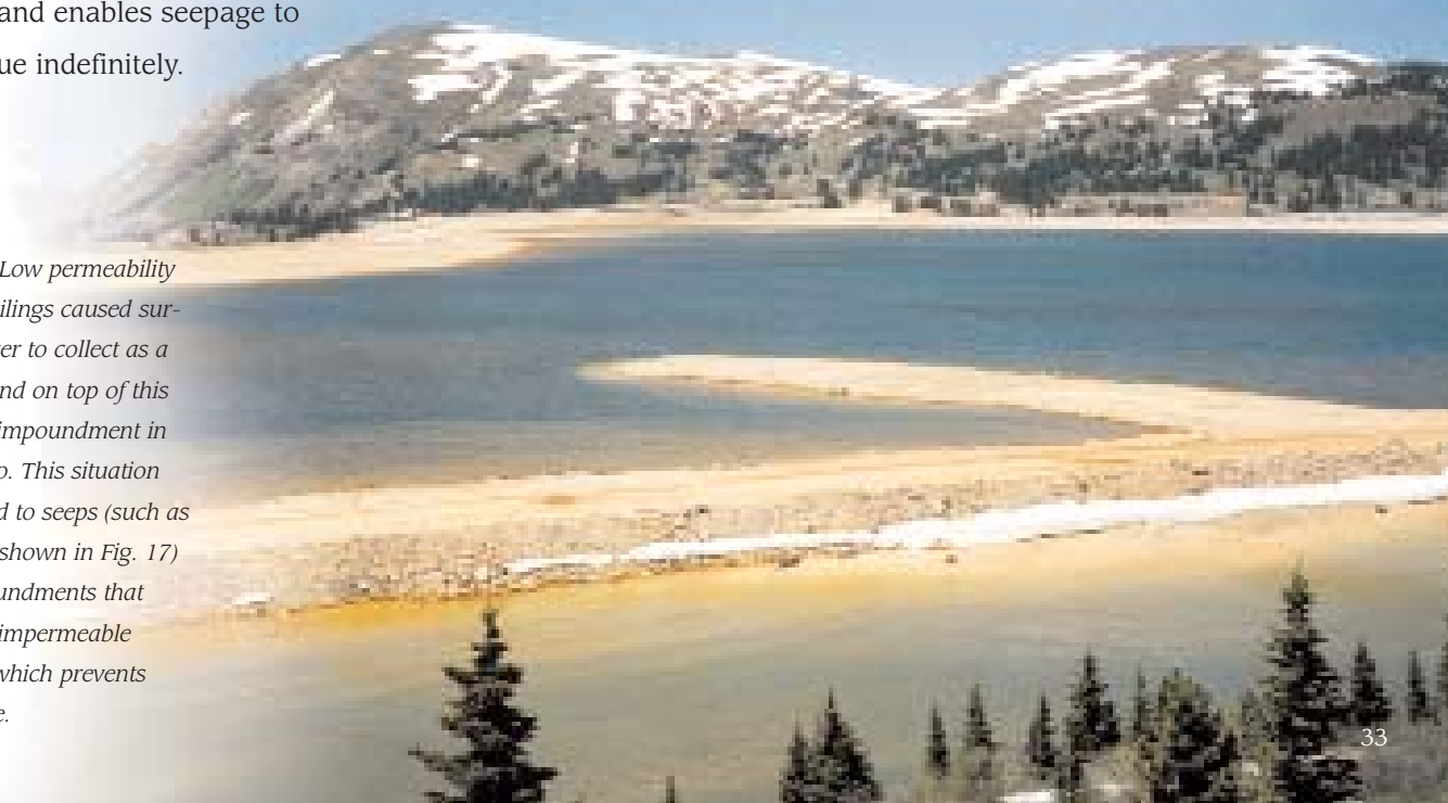
Fig. 17. Metal-bearing waters seep from the base of a mill tailing impoundment along Silver Creek in the Rico mining district of southwest Colorado.
