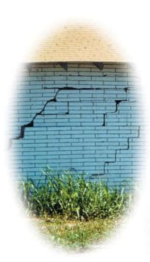
Fig. 15. Cracks in brick wall resulting from the failure of a foundation, caused by soil with a high content of expanding clays (D. Williams, NRCS, retired).
