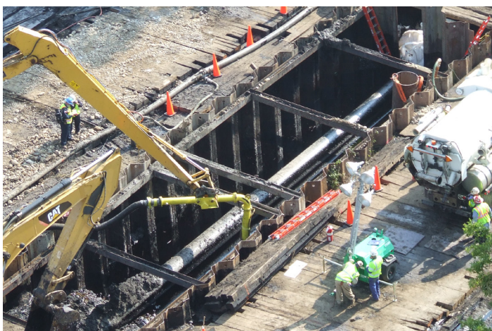
The damaged portion of Enbridge Line 6B is prepared for removal, having spilled hundreds of thousands of gallons of heavy crude oil near Marshall, Michigan, in July, 2010. Image credit: U.S. Environmental Protection Agency. 32
